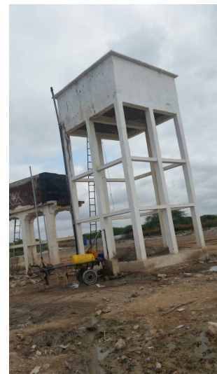
Water reservoir in Bardale, rehabilitated through public works
