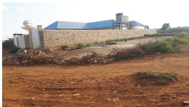
Perimeter Wall around the Towfiq MCH in Baidoa
