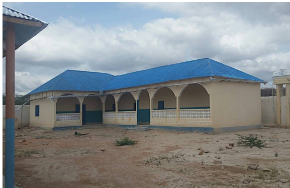
Administrative Block constructed in Bardale
