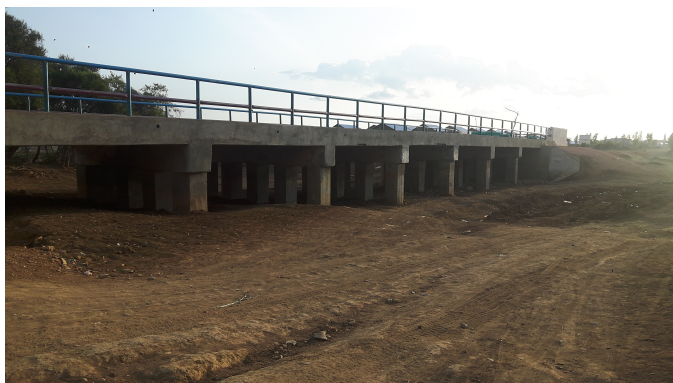
Rehabilitated bridge in Baidoa
