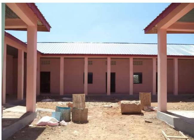
Rehabilitated building in Xudur with final supplies
