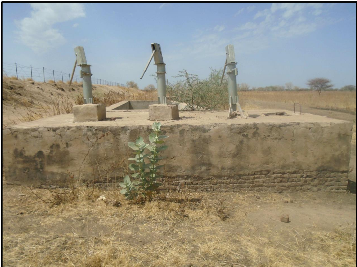
Picture 1: Three broken boreholes in Roshuk, Upper Nile State
