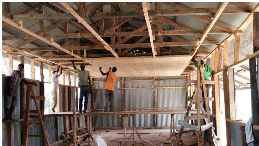
Photo 2 Construction team putting the ceiling for a shelter for returnees
