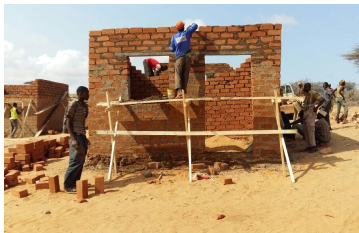
Photo 6 Building under construction
