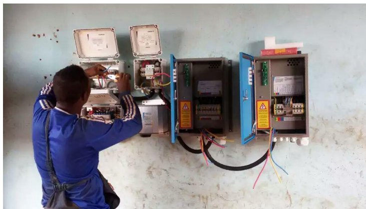
Photo 7 Electrical technician repairing fuse box
